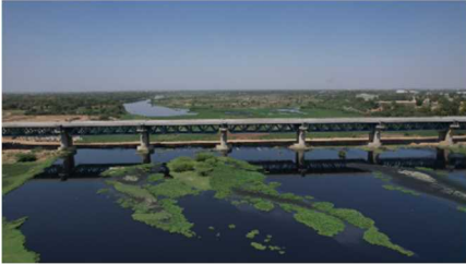
Sabarmati River Bridge
