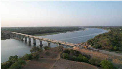
Mahi River Bridge
