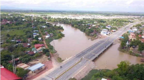
Completed Road Bridge
