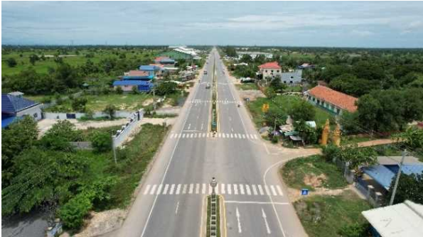
Completed Road (Rural Area)
